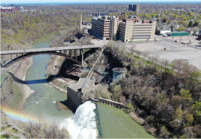
Station 5 powerhouse (top) at 103 Seth Green Drive, and aerial views from south (middle and bottom).
