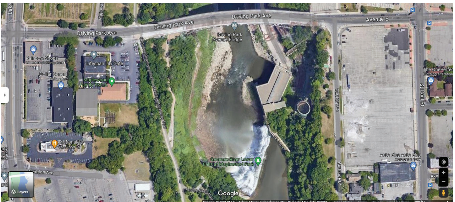
Station 5 aerial view.
