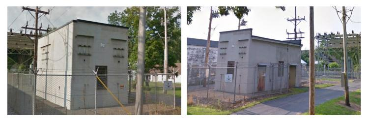
A new Control House will be built (at a different location within the property) featuring upgraded gas-insulated switchgear (GIS) technology and an updated control system. Additionally, a new and more efficient transformer will replace the current outdated version that has been in place since 1966, thereby providing more capacity and resiliency.
