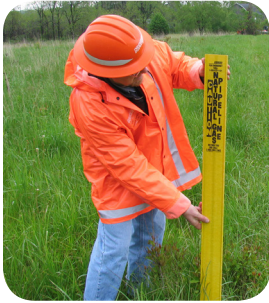
Line markers, such as the one above, indicate a buried natural gas pipeline's general location.
