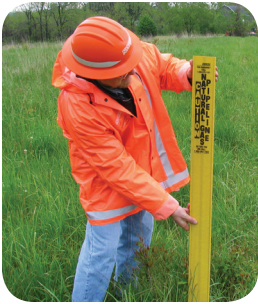
Line markers, such as the one above, indicate a buried natural gas pipeline's general location.
