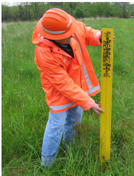
Line markers, such as the one above, indicate a buried natural gas pipeline's general location.
