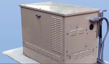
Typical stationary natural-gas fired generator
